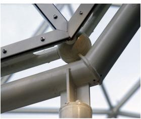
This pavilion in a park in Haarlem has originally been designed in 1984. The dome has a diameter of nine meters and is supported by ten columns. The design is based on the principle of a geodesic dome: a three frequency isosahedron. White powder coated aluminium bars and spheres make up the structure. The design has been awarded the first Aluminium Award in 1986. The triangular glass panels are placed on OTprofiles and are connected with aluminium screw strips.
