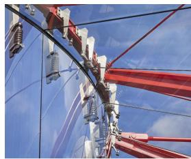
Octatube refurbished the concave suspended glass façade of London's Grade II-listed Channel 4 building, originally designed by Richard Rogers. With minimal modifications to the original design and with focus on reusing materials to minimise carbon footprint. The result respects the 1990's icon heritage. We have conducted structural assessments, calculations, and dismantling tests to understand the structural behaviour and condition of the façade.
