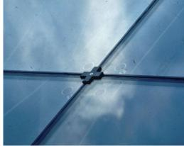
For the Fraunhofer Institut in Darmstadt, Octatube was responsible for the design, engineeirng, production and installation of a structural facade, an atrium roof light and the canopy above the main entrance. The structural facade has large glass panels that are fixed to a very slender construction of cables and tension rods by means of Quattro nodes. The atrium roof light is constructed of ultra light tensile trusses. Here, the double glass units are fixed with a structural bonding.
