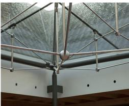
The architect (Van Hoogevest Architecten) was commissionned to design a restorationplan for the castle & coach house and a newly built care centre. For the castle Octatube has done the engineering, production and assembly for a 60 m2 skylight with stainless steel tension bars.
