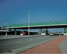
In the eighties, the young architectural firm Benthem and Crouwel was assigned to design several customs emplacements. The aim was to realise recognizable, uniform and flexible structures. The spaceframes that were developed by Octatube proved to be a suitable system for these preconditions and the construction of suspended roofs.
