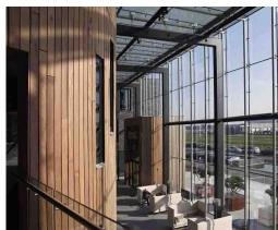
The interior space of the DMG atrium is a generous entrance area and informal meeting place that seems to have an open connection to the exterior. This large connecting atrium between two offices is designed as Quattro façade with a bonded point-fixed connection of the glass. In the atrium are five large rectangular portals. From these portals, air is blown into the atrium. On top of the portals round tubes are placed that support elliptical shaped secondary steel portals.
