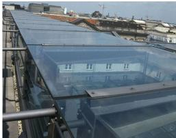
The double glass façade for the Deutsche Guggenheim (Unter den Linden, Berlin) was designed by architect Novotny & Mähner in order to smoothen out the difference between the existing stone façade and the new double steel/aluminum topping up by a reflection. The glazing was monolithic clear fully tempered glass with stainless steel frames as projections of the existing window scheme. The glass and profiles are suspended from brackets at the roof top.
