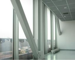
The Hollander project in Barendrecht is an extension of the Greenery distribution centre with a new head office, pilotage office and shipping office. As an alternative to aluminium, a steel window frame with four-sided surface mounted glass is preferred for the entire façade surface.
