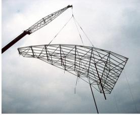
For a large dome covering a swimming pool a spaceframe in the Tuball system has been applied. The structure has a diameter of 50 meters, and a minimal geometry of intertwined delta beams. The steel spaceframe is galvanized and powdercoated, including the bolted connections. This has been done in order to prevent corrosion in the swimming pool environment. The construction has been cladded with insulated glass units, fixed on aluminium skylight profiles.
