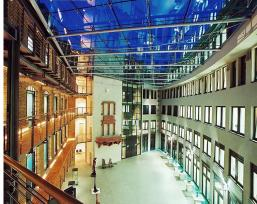
The Haus des Handwerks is a complex of redeveloped buildings. The open space in between the buildings has a complex floor plan and has been covered by a transparant glass roof on a filigrain steel construction. This atrium is supported by four meters long round stainless steel bars with a 3D tensegrity truss underneath. Half of the stainless steel cast glass-nodes are attached with an adjustable screwed connection.
