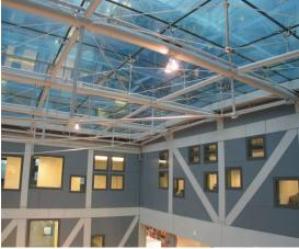
The FBOR building in Groningen is a new development of the University of Groningen Faculty of Mathematics & Physics. Two atriums with skylights are situated in the building. The biggest skylight has a span of 26 meters. On the long side the roof is executed with subtend beams.
