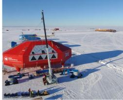
Octatube developed in combination with Hugh Broughton Architects in London two glass cockpits for the British Antarctic Survey. The cockpits will be used as panoramic viewpoints for the red Module A. They are constructed of a steel frame with warm bend insulated glass units sitting on top. The panels are structurally silicon bonded and are designed to withstand temperature differences up to -55°C and wind gushes of 300 km/h.
