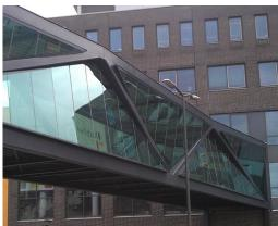
The main building (2008 - AGS Architekten & Planners) and the extension by LIAG Architecten is connected on the first floor by a bridge of steel and glass, spanning 40 meters. The irregular structural steel lattice is filled in with 122 unique single glass planes tilting forward and backward emphasizing the triangular form language.
