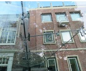
The entrance of Noord-Holland's State House (also known as the Dreefgebouw) parking garage is marked by a full glass entrance. This glass structure is feature by laminated glass panels that are interconnected by means of high-end duplex stainless steel nodes. Some glass units act as a portal, while the entrance facade itself functions as a three-hinged glass arch.
