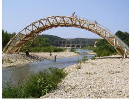
The temporary cardboard bridge near Avignon in the south of France, has a span of 20 meters and is build up by 280 cardboard tubes, each with a diameter of 115mm and a thickness of 19mm. The steps are made of recycled paper and plastic. The bridge has been exposed to the public for 2 months during a cultural event. It is located only a short distance away from the famous Roman aquaduct the Pont du Gard in France. The cardboard structure has been installed and disassembled again several summers.
