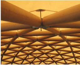
The Paperdome was the first cardboard project collaboratively executed by Octatube and architect Shigeru Ban. Choreographer Jeanette van Steen initiated the project by asking architect Shigeru Ban to design a temporary theater. The Japanese architect designed a dome with a span of 30 meters, based on a 10-frequency subdivision and consisting of cardboard tubes. It was produced and installed in IJburg (Amsterdam) in the spring of 2003 within 7 weeks.
