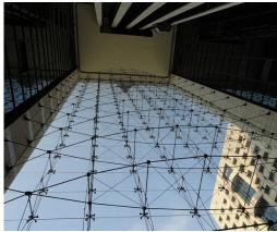
Quattro nodes provide the interface between the glass sheet and the stabilising support structure. The form of the nodes is derived from the shortest distance between the holes in the glass sheet and the central placement of the support structure, which normally runs along the axis between two glass panels. With four holes in the corners of each of four glass panels, the typical resulting form is a diagonal cross.
