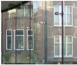
When it comes to all-glass structures, the most commonly used elements are glass fins. These building components utilize the full potential of glass as a structural material, and at the same time yield maximum transparency and an unobstructed open view. Glass fins eliminate the need for conventional metal mullions and beams. In facades and roofs the glass fins can be structurally used to transfer horizontal and vertical loads from e.g. wind and snow to the structure.
