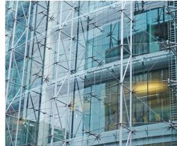
The architectonic aim of Octatube's utilization of glass, is to deliver surfaces with maximal transparency, preferably by maximizing the self supporting capabilities of glass, creating slender and elegant structures.
