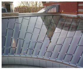
MUMA Architects, Dewhurst Macfarlane Engineers and Octatube designed a spectacular glass roof that rises 14 meters above a new gallery floor. The 73 laminated heat-strengthened glass beams, spanning up to a maximum length of 11m. The surface of the roof is formed by insulated glass panels that are fixed by point connectors in the glass seams and a continuous stainless-steel profile on top of the glass beams. The total area of the glass roof is approximately 370 square meters.
