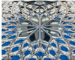
A new and contemporary pavilion has been realised in the Grand Courtyard of The OWO, the former Old War Office in Whitehall, London. Mirror-polished 3D stainless steel panels on the roof give the pavilion its striking appearance. Octatube translated the highly bespoke design of this pavilion into a technical proposal, and was appointed to engineer and built it. The extraordinary geometry of the pavilion has no straight lines and therefor required bespoke solutions and clever craftmanship.
