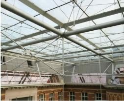
The main load bearing construction of the roof over this atrium, 26 by 28 meters, consists of a constructive grid of intersecting tubes in two directions. Maximal module size is eight by eight meters. These tubes are fitted with round tension trusses for vertical downward forces and vertical compression tubes on the intersection of the large tubes.
